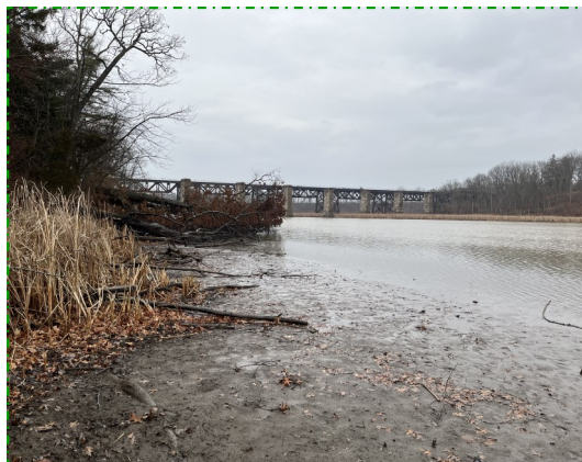
Train trestle over Twenty Mile Creek in Jordan Station . © Bob Highcock
